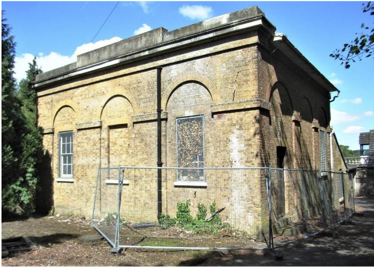
C Amwell Hill pumping station
