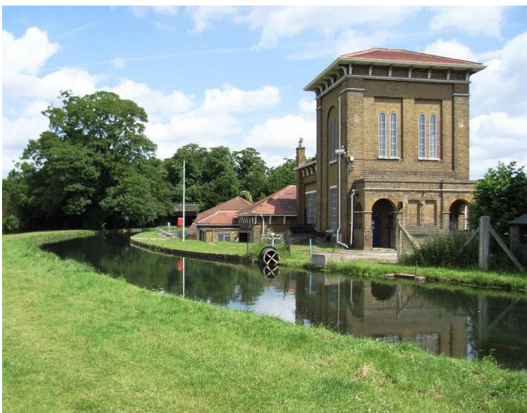
E Rye Common [St Margarets] Pumping Station
