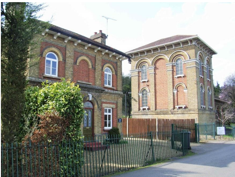
D Amwell Marsh pumping station
