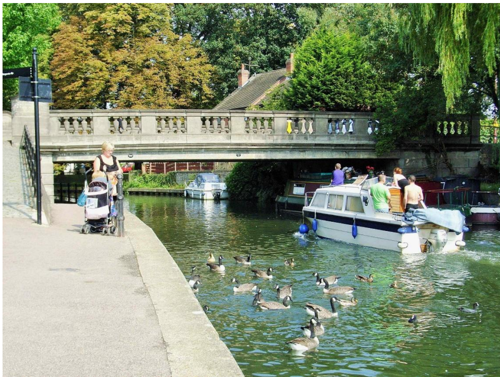
A 2011 view of the bridge showing the river being enjoyed by humans and ducks alike. The bridge provides a headroom clearance of nine feet six inches during normal river conditions.
